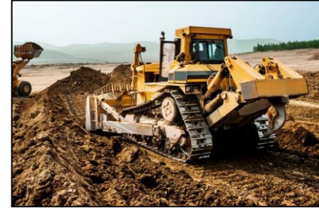
Excavation – lot grading, street excavation and utility work currently underway
