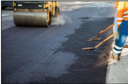
Street Paving – streets are currently being poured, but are not accessible
